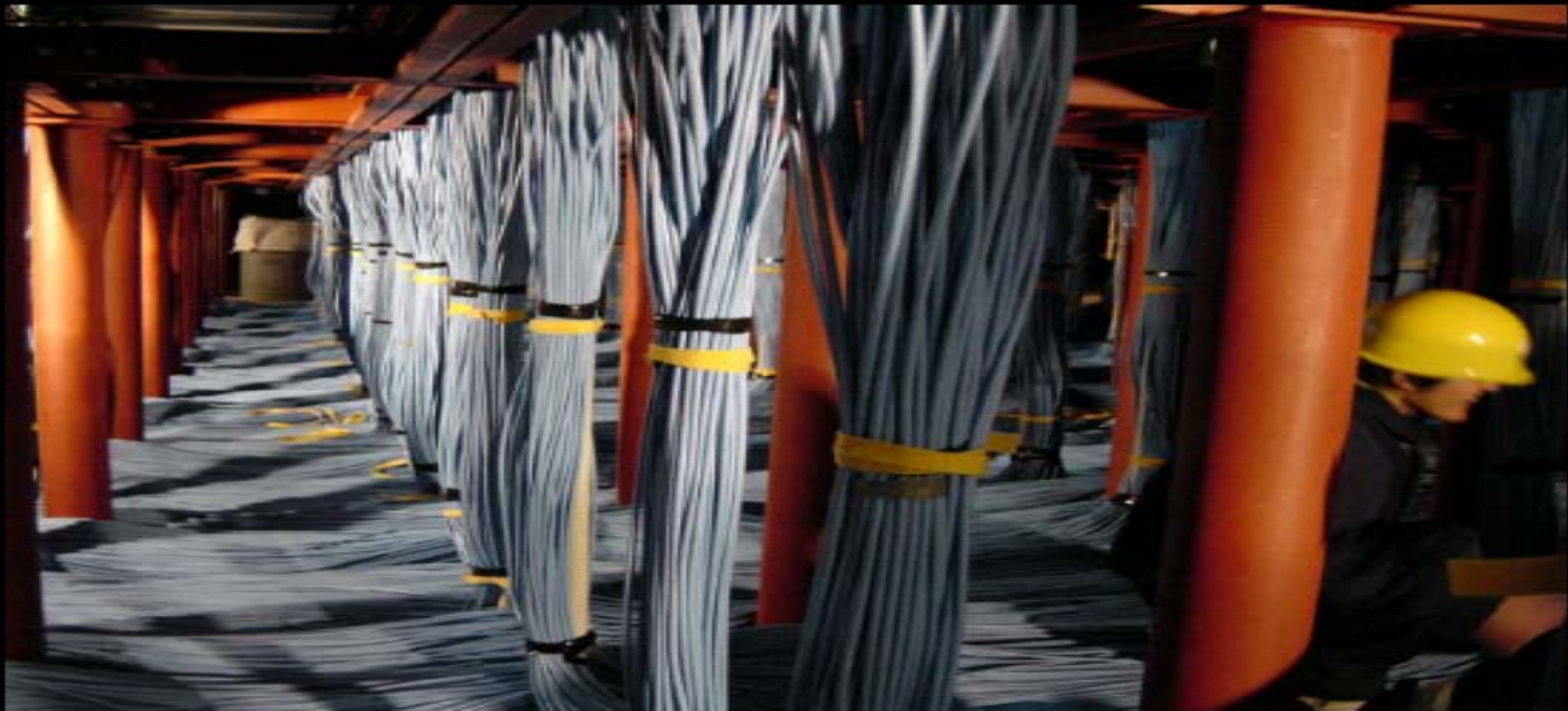
Wiring of interconnection network cables
